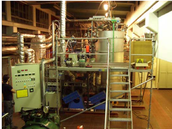
Figure 1: Front side of the Chalmers 100 kW oxy-fuel combustion test unit showing top fired 3 meters high combustion
